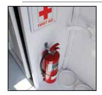
20-pound ABC dry chemical fire extinguishers are provided in all chambers. Mounted and secured inside the airlock compartment and/or placed beneath the seats.
